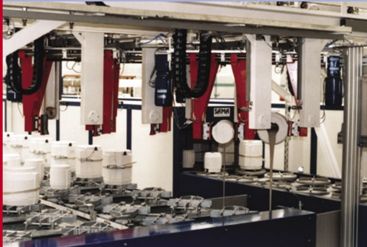
HOHLGESCHIRRGIESSANLAGE HOLLOW WARE CASTING PLANT
